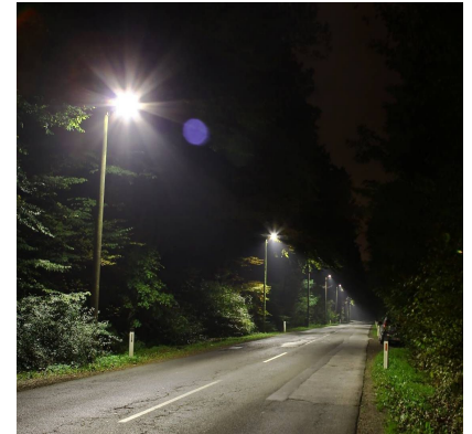
Lamp after reconstruction
